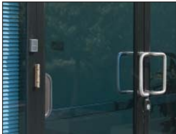
Detachable antenna unit shown mounted away from the control unit.
